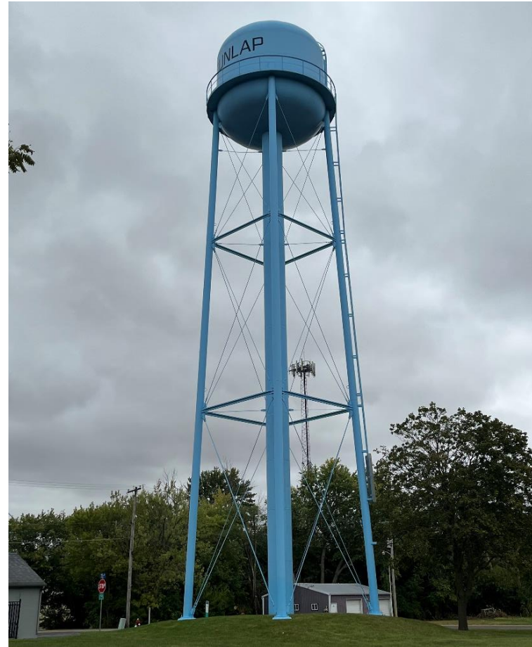
Figure 23: Dunlap Water Tower
