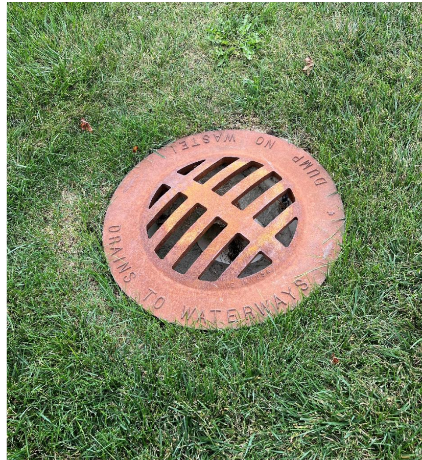
Figure 25: Dunlap Stormwater Drain
